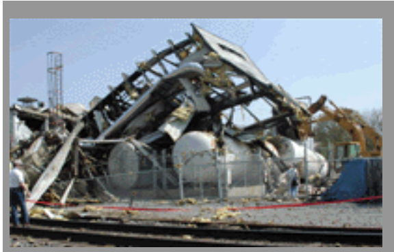
This accident investigated by and picture provided by the U.S. Chemical Safety and Hazard Investigation Board. Visit their site at http://www.csb.gov
