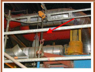
This picture shows an improvised pipe support made from scaffolding, springs and clamps.
