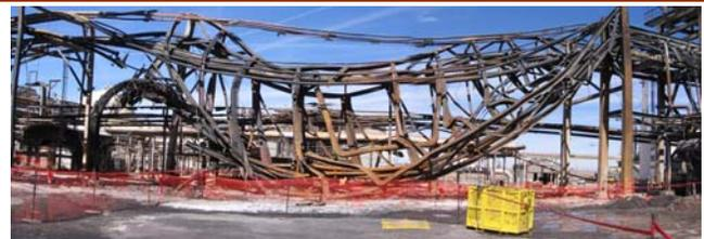
***Is your unused piping and equipment disconnected or positively isolated?***
