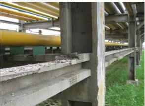
← Some examples of damage to fireproofing on steel pipe bridge supports – the fireproofing has been removed, or has become degraded and fallen off.
