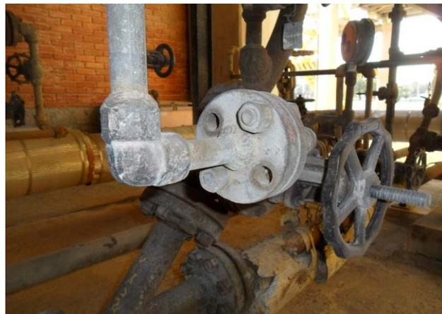
The pictures show improperly bolted flanges that a plant found during safety inspections. In the top pictures, some or all of the bolts are too short, and the nuts are not completely on the bolts. This means that the joint may not be as strong as it should be. Flanges are designed so that the entire nut-bolt combination holds the forces on the flange. If the nut is only partially screwed onto the bolt, the connection may not be strong enough.
