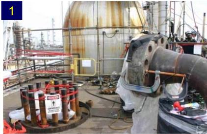
A maintenance crew was re-installing piping at the top of a reactor in a refinery. The reactor was being purged with nitrogen to keep oxygen in the air from contacting the catalyst inside, and the top of the reactor was open (1). A sign indicated that the reactor was a confined space and a permit was required for entry, but no sign warned about the presence of nitrogen. On the job permit, the box indicating “Nitrogen Purge or Inerted” was checked “N/A” – Not Applicable (2).
