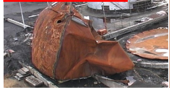
Fig.2 : Hot oil tanks
