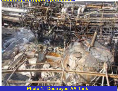
Photo 1: Destroyed AA Tank
