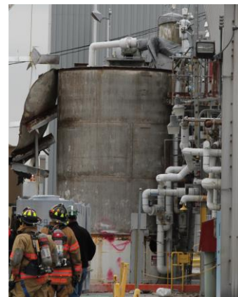
Aftermath from a fatal fire and overpressure during hot work.
