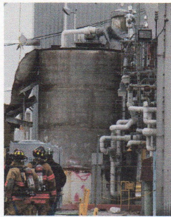
Aftermath from a fatal fire and overpressure during hot work.
