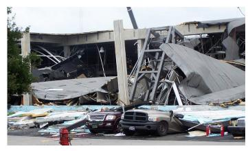
What happened? On June 9, 2009, a natural gas explosion damaged a meat processing factory in Garner, North Carolina. Three workers were killed when a section of the building collapsed. Four workers were critically burned, and 71 persons were sent to the hospital. Three firefighters were exposed to toxic anhydrous ammonia from the plant's refrigeration system. About 18,000 lbs (8165 kg) of ammonia were released and a large area of the plant was damaged.
