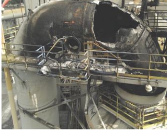
Fig. 2: After the fire
