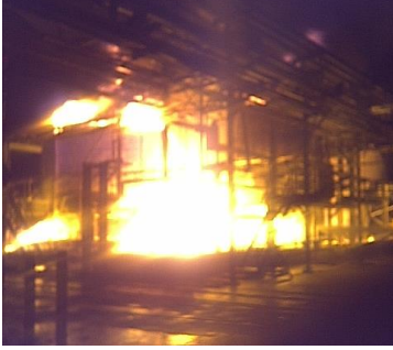
Figure 1. Tanks ablaze after a lightning strike
