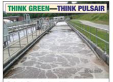
Pulsair Chemical and Wastewater Mixing Systems efficiently mix aeration tanks, anoxic basins, sludge tanks, and chemical tanks using up to 75% Less Energy than conventional mechanical mixers...and there are no immersed impellors, shafts, gears, seals or any other moving parts in the tank.
