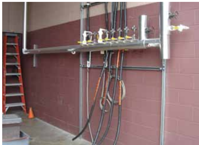
▲ Figure 4. Pretraced and insulated tubing bundles connected to a steam feed manifold make for a much smaller and neater installation. Simply remove the bundle from a roll, then connect it to the process and to the tracing supply and return.
