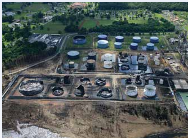
▲ The tank farm incurred significant damage.
