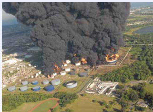
▲ Multiple tanks caught fire during the incident.
