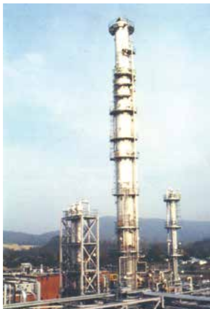
▲ Figure 2. Eastman's methyl acetate process combines multiple steps into one column by applying process intensification. The reactive distillation column is located at Eastman's chemicals-from-coal complex in Kingsport, TN. Image courtesy of Eastman, all rights reserved.
