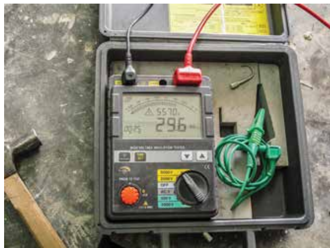
▲ Figure 2. A megger check tests the insulation resistance of both the cable and power wires to isolate potential faults to ground.
