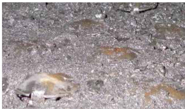
▲ Figure 1. Electrolyte modeling tools can be combined with process simulators to predict fouling and corrosion conditions in crude distillation towers. The photo shows a distillation valve tray with severe scaling and fouling. Image courtesy of Doug Bouck.
