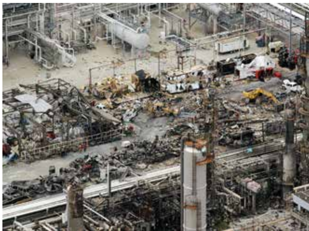
▲ Figure 2. A risk-assessment team violated company risk-management procedures and siting criteria when they allowed temporary office trailers to be placed in close proximity to hydrocarbon processing units that were temporarily offline. During startup of the units, an incident occurred that killed 15 workers in the nearby office trailers. Source: (4).
