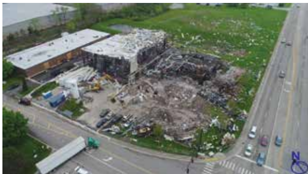
▲ A hydrogen explosion occurred during a mixing procedure. Read U.S. Chemical Safety and Hazard Investigation Report No. 2019-03-I-IL for more information.
