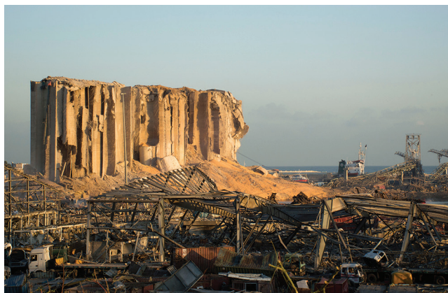
▲ Figure 4. The Beirut Port incident that took place August 2020 was the result of the explosion of 2,750 kg of ammonium nitrate.
