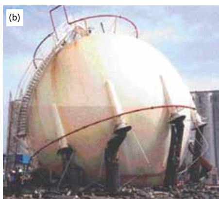
▲ Figure 1. Corrosion has been the cause of many past process safety incidents. Image (a) adapted from U.S. Chemical Safety and Hazard Investigation Board (CSB) Report No. 2012-03-I-CA.
