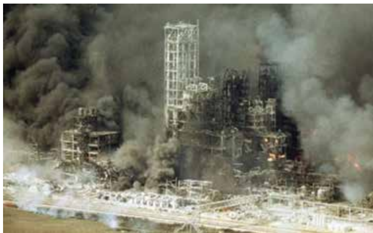
▲ Figure 1. In 1989, a fire at a plastics plant in Pasadena, TX, began after operators bypassed proper maintenance procedures. The ensuing fires took 10 hours to be brought under control (1).
