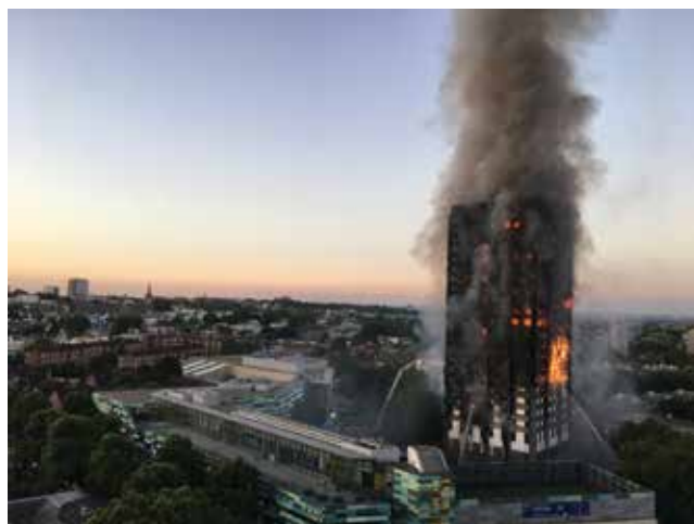
▲ Figure 3. The Grenfell Tower fire resulted in catastrophic loss of life and property in 2017. During a building renovation project two years earlier, the building's cladding was replaced with materials that were less expensive than the original cladding, which reduced the structure's fire resistance. Image courtesy of Natalie Oxford (2017).
