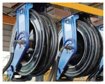
▲ Figure 1. During a safety audit, an individual noticed that two identical hose reels were used for two entirely different processes, and accidentally using one hose for the wrong process would end in a serious safety incident. This hazard would not have been resolved if it were not for one individual speaking up.
