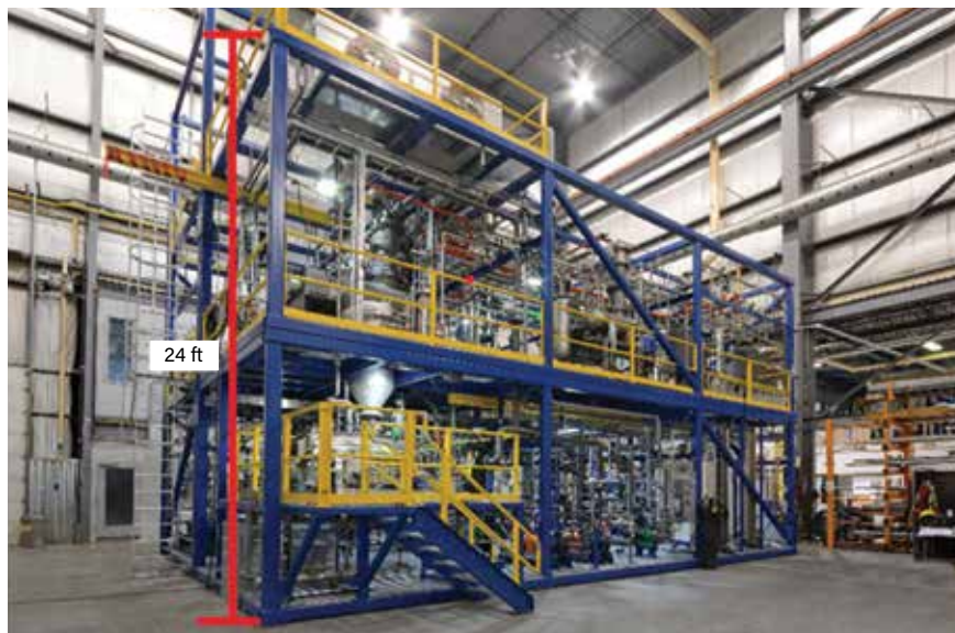
◀ Figure 3. A pool fire scenario, in which a large quantity of liquid fuel collects and ignites, can span more than 2,500 ft 2 (30-ft radius) and reach more than 24 ft in height.
