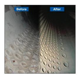
One old "Best practice" involved maintaining a thin scale on boiler tubes in order to minimize offline oxygen corrosion!!
