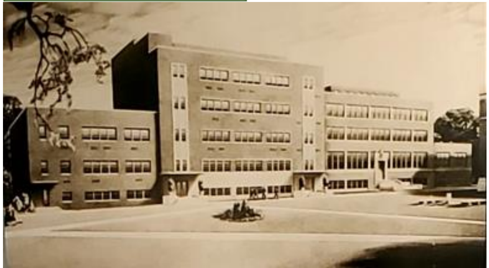
AW Smith Building (west elevation) for CWRU Chemical Engineering
