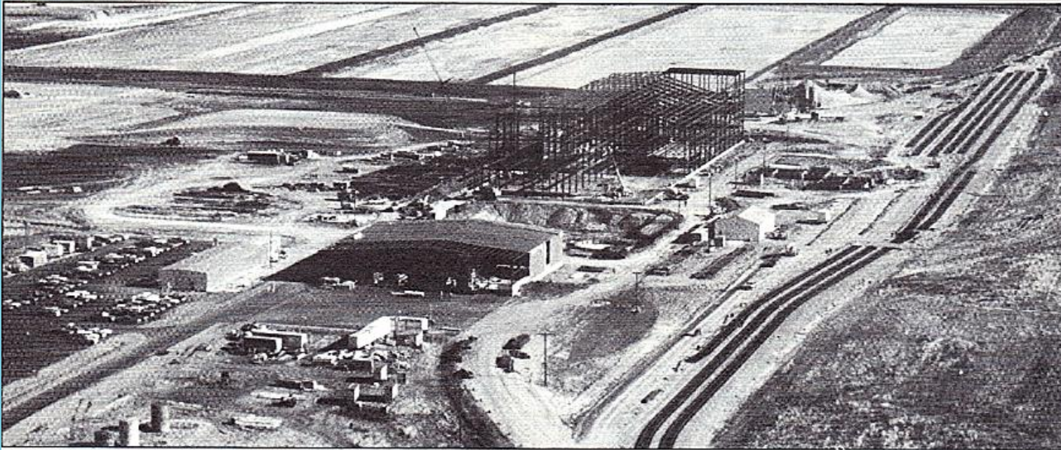
$43-MILLION BEET SUGAR PLANT — A Project in Progress
