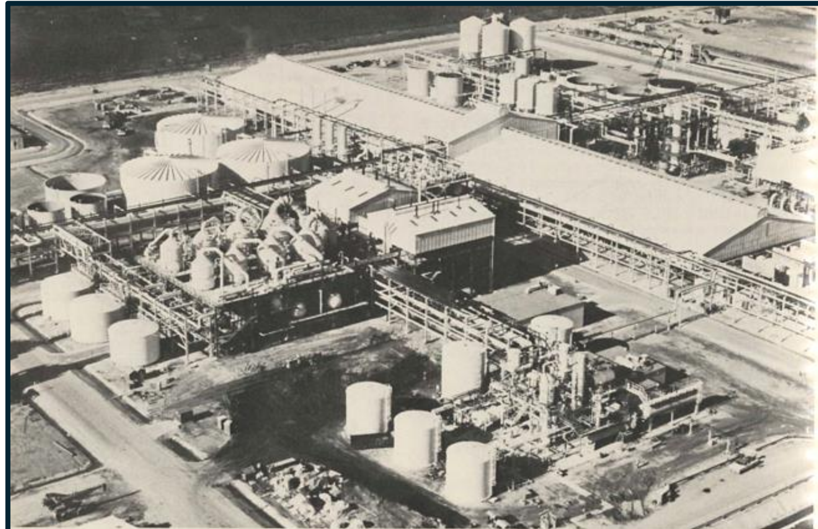
Diamond Shamrock's Battleground Plant in Houston, Texas. 5
