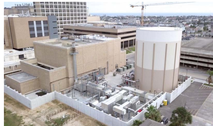
The UTMB CHP systems protected by a flood wall, photos courtesy of Affiliated Engineers
