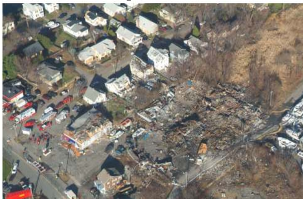
CONFINED SPACE EXPLOSION Danvers, Massachusetts November 22, 2006
