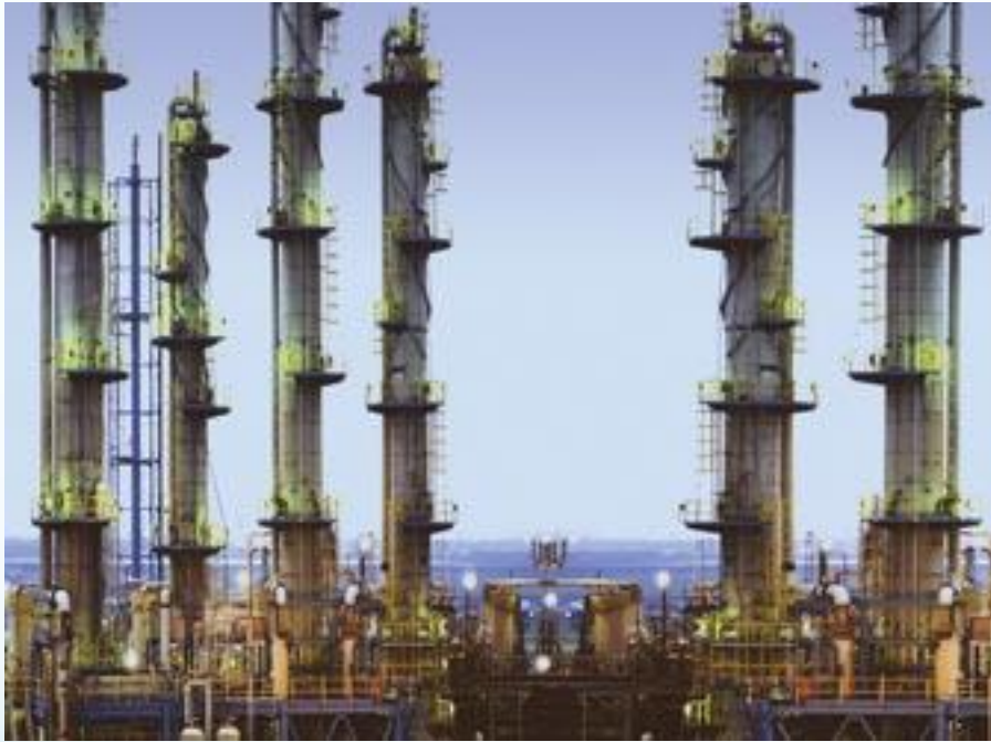
Fractional distillation columns at an oil refinery
