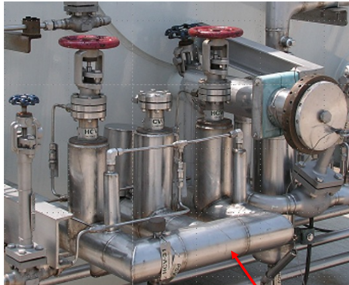
Vacuum Jacketed Fill Pipe
