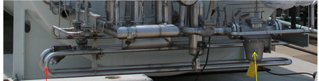
Pressure Build Regulator PCV-1
