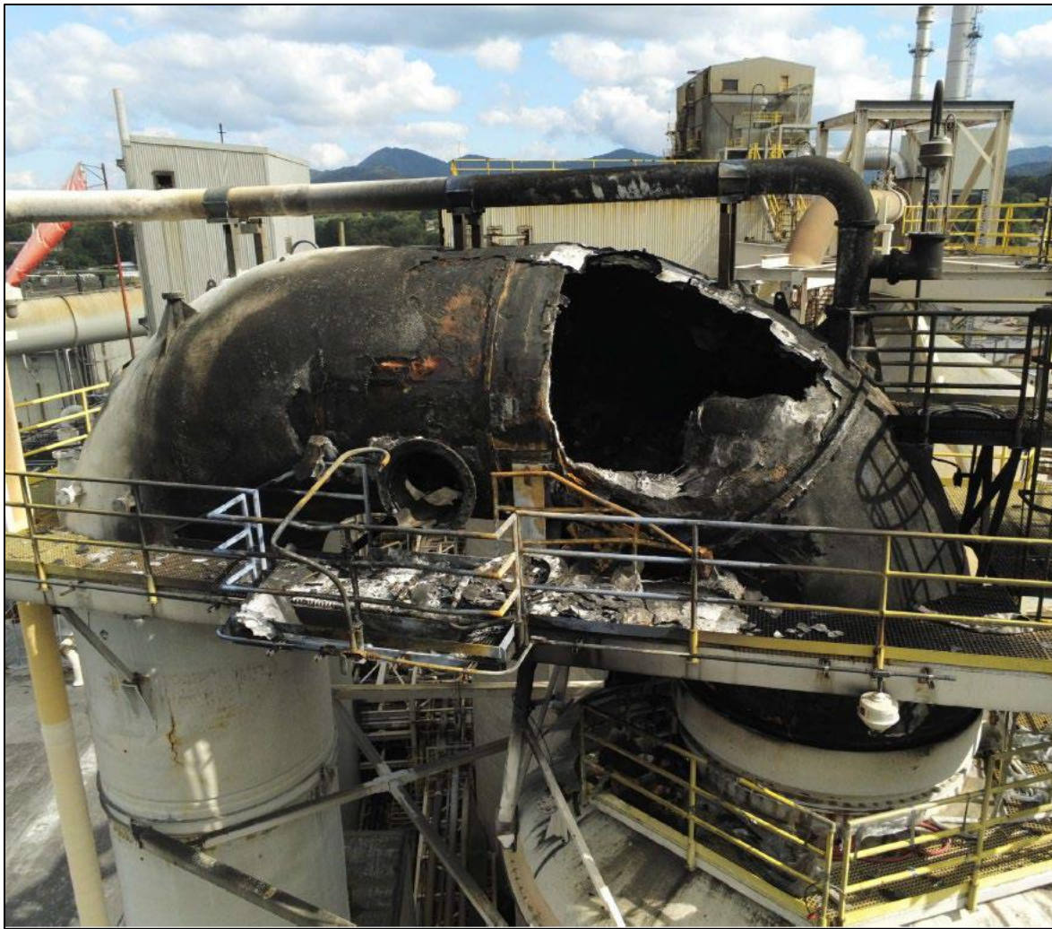
Figure 2: Fire damage at Evergreen Packaging upflow (left) and downflow (right) towers. The fatally injured workers were in the lower portion of the downflow tower and were prevented from reaching the emergency egress point by smoke and flames. The egress location is the manhole located at the bottom of the arch. [2]
