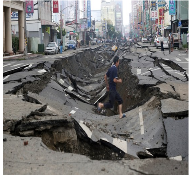
July 31 st Taiwan: propylene pipeline explosion
