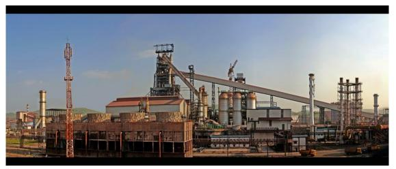
Modern Blast Furnace 100 feet tall 15,000 tons iron/day
