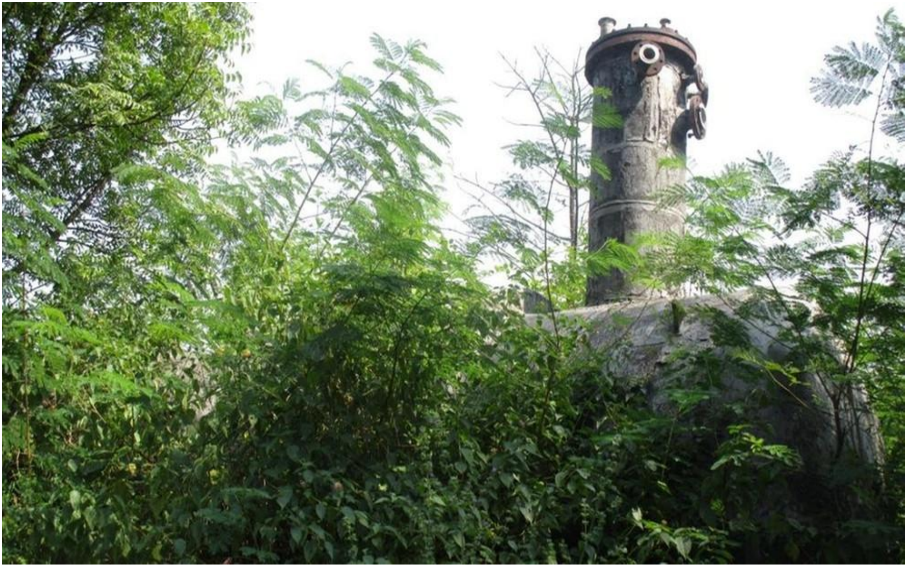
Tank 610 which contained 40 tons of MIC
