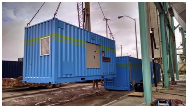
Figure 14. Unloading the ECL system at the PacifiCorp Power Station in Wyoming
