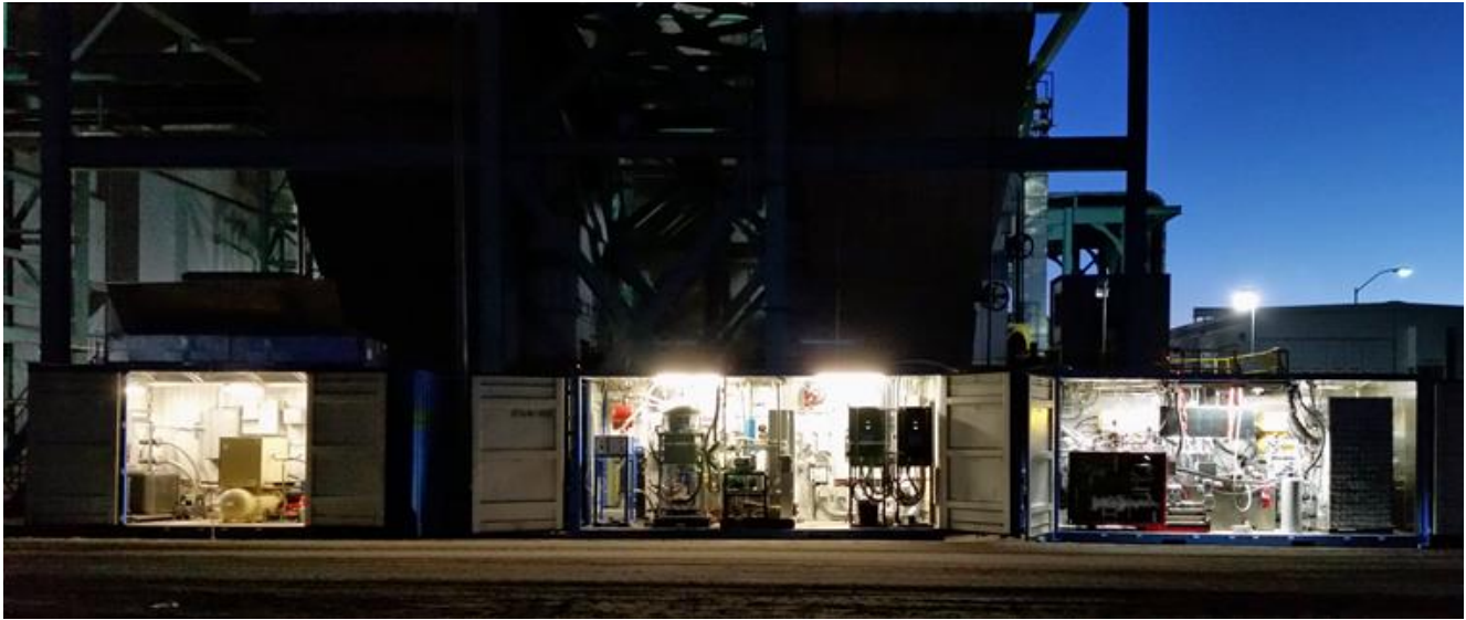
Figure 15. Testing the ECL on Unit #3 at the Power Station
