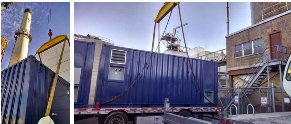
Figure 8. CCC-CFG™ system being unloaded at BYU Heating Plant
