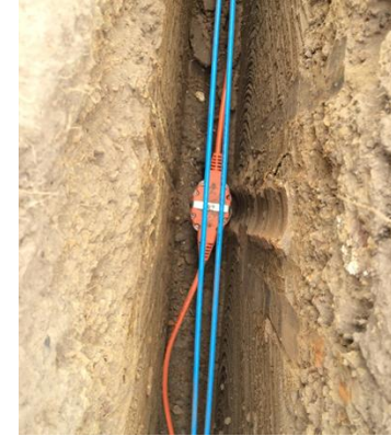
Deployed in trench
