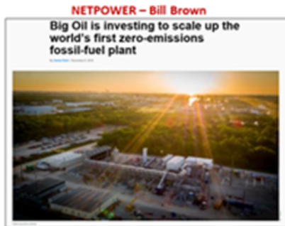
CO 2 Plant Capture
