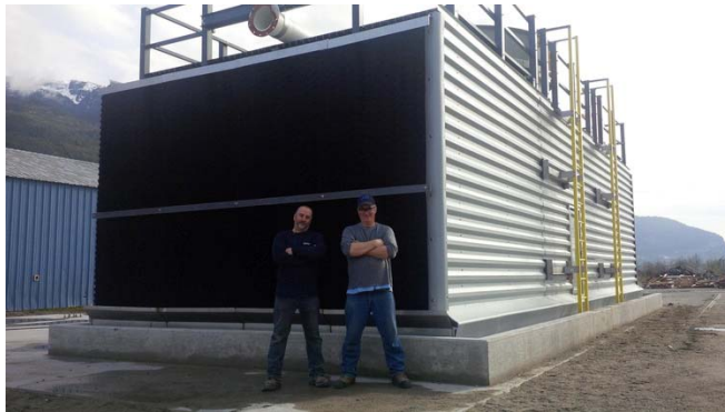
Squamish demo plant site construction
