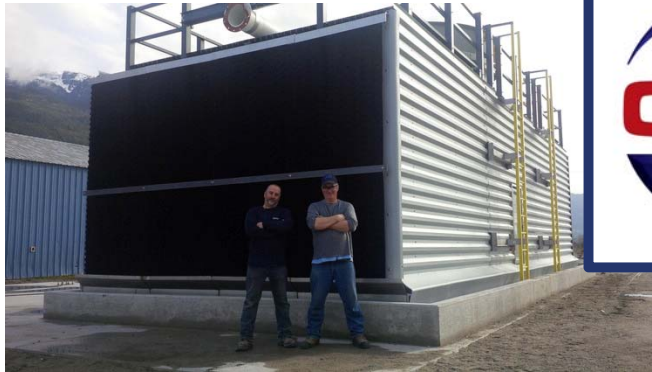
Squamish demo plant site construction
